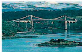
мост most bridge
